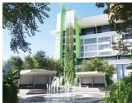
ATIVO PLAZA DAMANSARA AVENUE MALAYSIA
