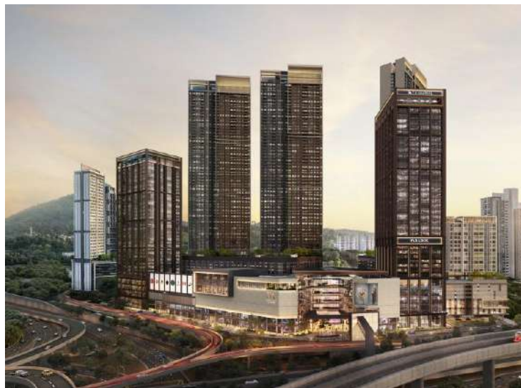
ATIVO ANNEXE @ DAMANSARA AVENUE MALAYSIA
