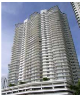
IDAMAN RESIDENCE KUALA LUMPUR, MALAYSIA
